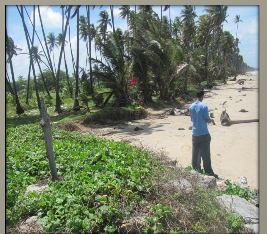
Flanking on northern end of north revetment
