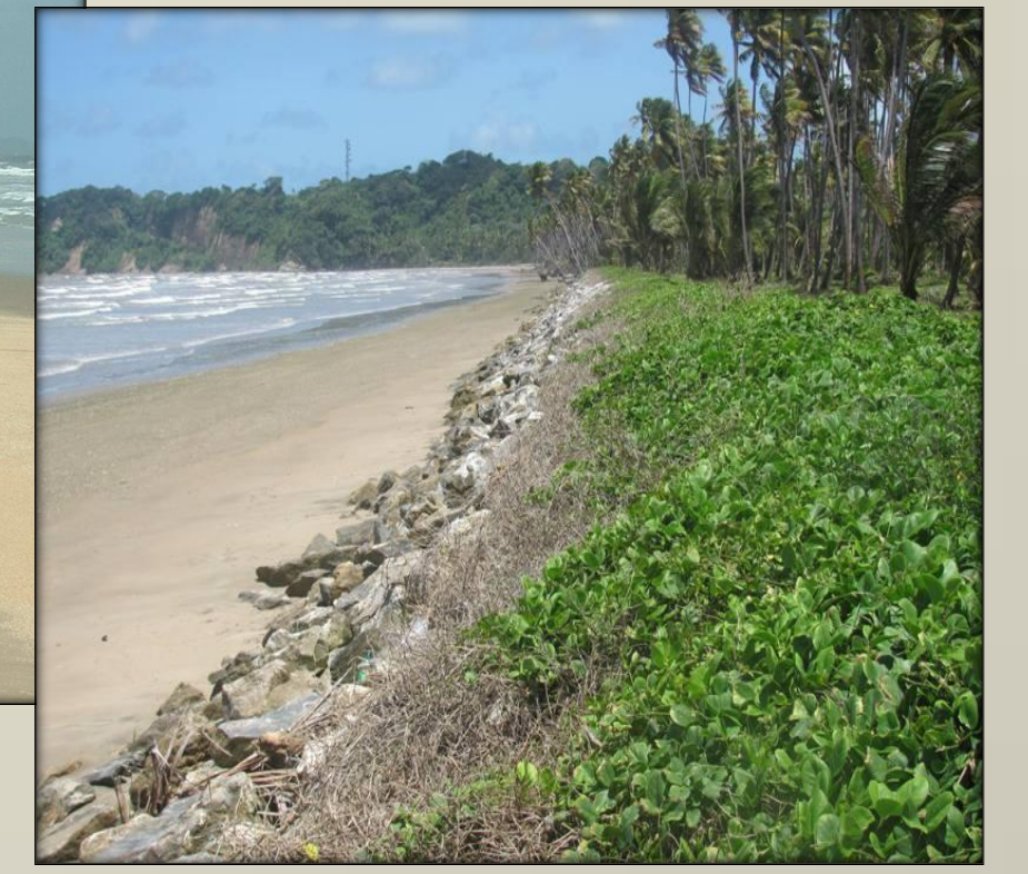
Revetment 6 years after completion
