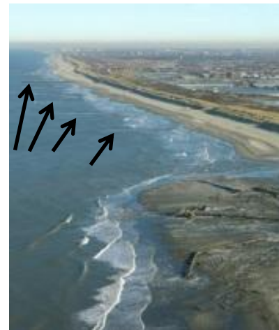
Figure 3: Aerial photograph of the northern end of the Vlughtenburg field site during construction. Groynes at the southern end are already covered with sand. (source: www.delflandsekust.nl )
