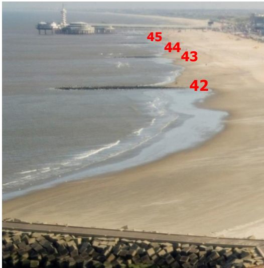
Figure 4: Beach of Scheveningen prior to the nourishment in 2009. Numbers correspond to individual groynes. (source: www.kustfoto.nl )
