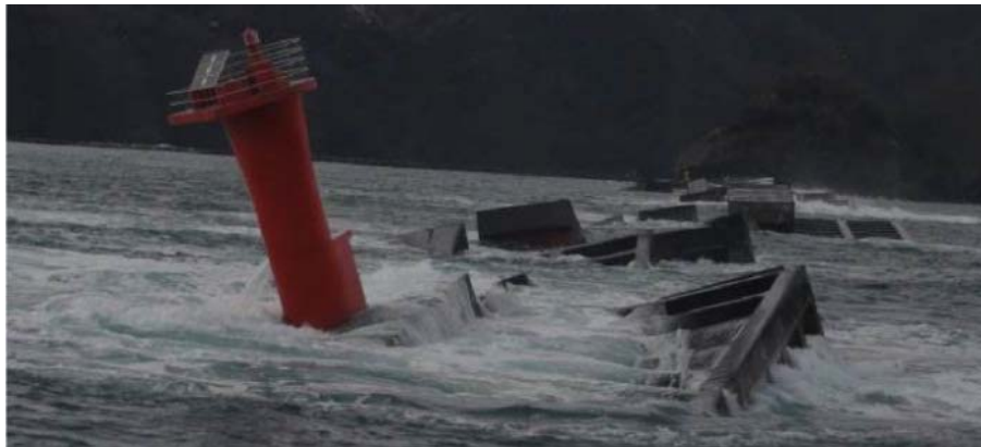
Photo 2. State of damage of North Breakwater
