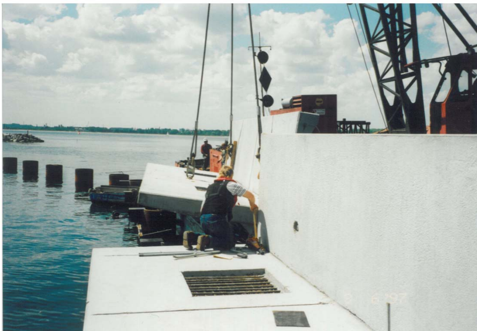
Figure 1. Breakwater Construction at Laboe, Baltic Sea, Germany
