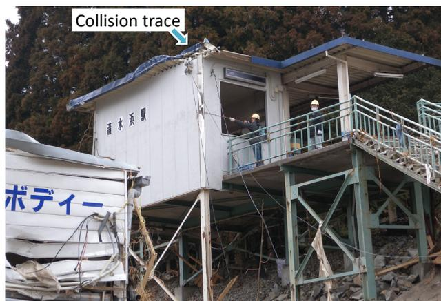
Photo 6. Tsunami traces on the building of Shizuhama Station (The photo was taken on April 3, 2011.).
