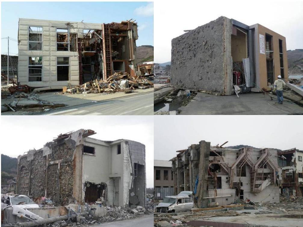
Photo 11. Examples of reinforced concrete buildings collapsed in Onagawa Town (The photos were taken on April 26, 2011.).
