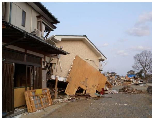
Photo 2. Damaged houses in Hajikamimukaibara, where the left-hand side house was collided with the second floor of the right-hand side house (The photo was taken on April 2, 2011.).
