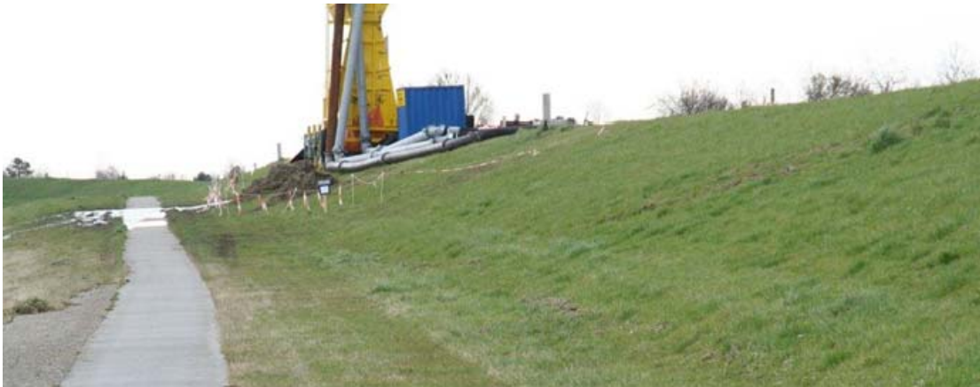
Figure 3. Typical Dutch sea dike: protected down slope, (partly) protected berm and grassed upper slope. This upper slope can be attacked by up-rushing waves.
