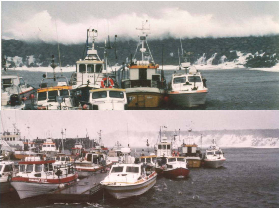
Figure 15. Rear side of the Bakkafjordur breakwater during a storm in 25 October 1995, overtopping over the crest and through the crest.
