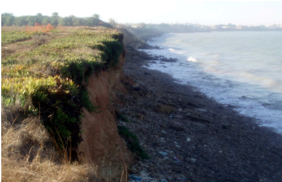
Figure 2 – Erosion of cliffs in Chipiona shoreline
