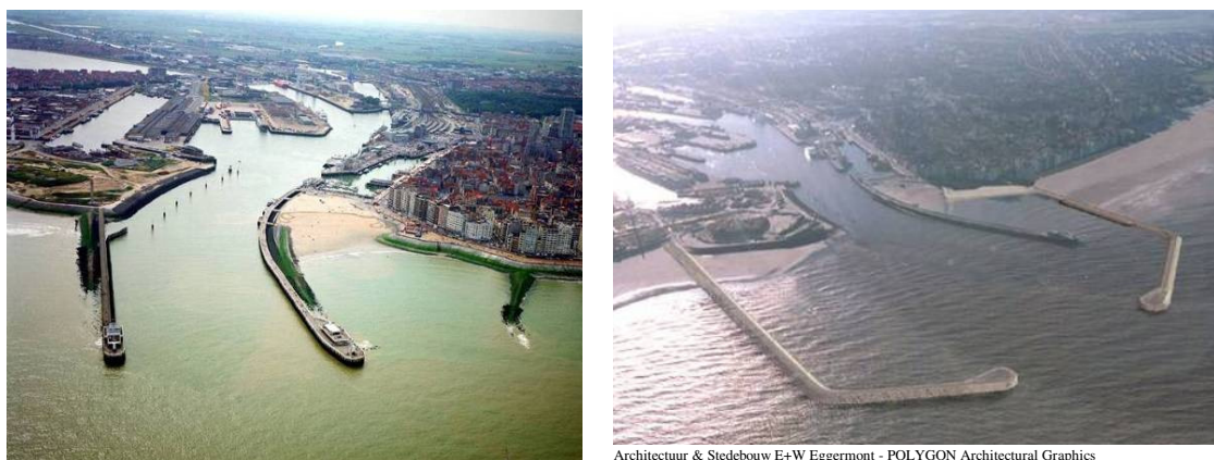
Figure 1. Old harbour access defined by two piers (left) - New harbour access with access channel perpendicular to the coast and two new breakwaters (right).
