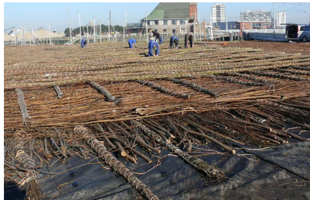
Figure 4. Construction of willow mattresses in Ostend.
