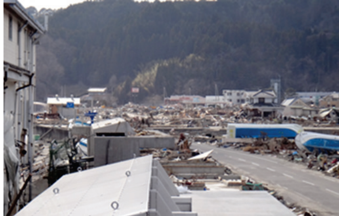
Photograph 2. View from top of the new seawall overlooking the Osawa Area of Yamada Town toward the old seawall section to the west. The old section was significantly lower with a height of 4.0m above MSL compared to the new 6.6m high section.
