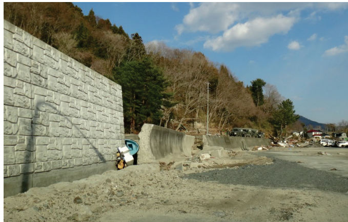
Photograph 4. Open end of the new seawall section at Osawa Area of Yamada Town. The old seawall at the transition was broken by the tsunami. The road passing through the opening leads to northern coastal villages on Omoe Peninsula.
