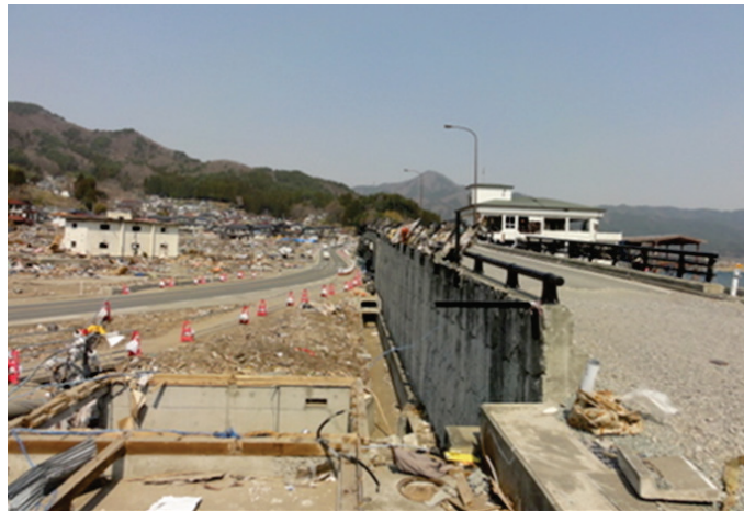
Photograph 8. Kirikiri Town flushed by the tsunami at the left. A tsunami trace at 16.2m was found on the roof of the seaward RC 4-story building.
