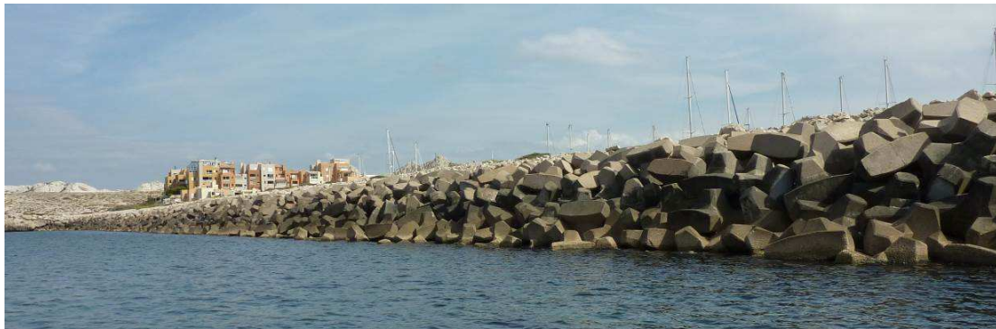
Figure 4. Le Frioul breakwater, in the South of France, built in 1984.
