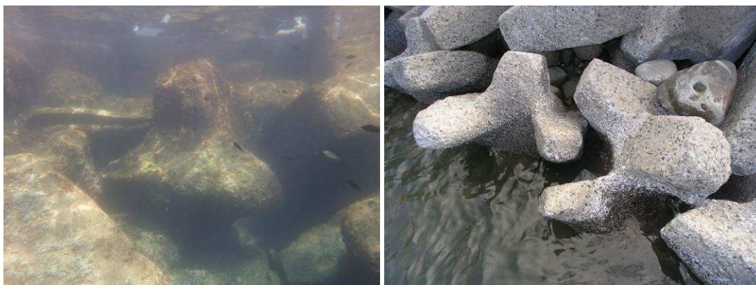
Figure 7. Unit not interlocked, rounded shape (left). Units worn out by mechanical action of the sand and small rocks projected by the waves (right).
