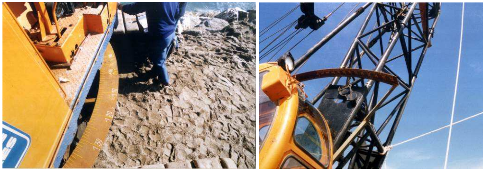
Figure 2. Compass frame welded on the crane (left) and frame for the vertical angle of the boom (right).
