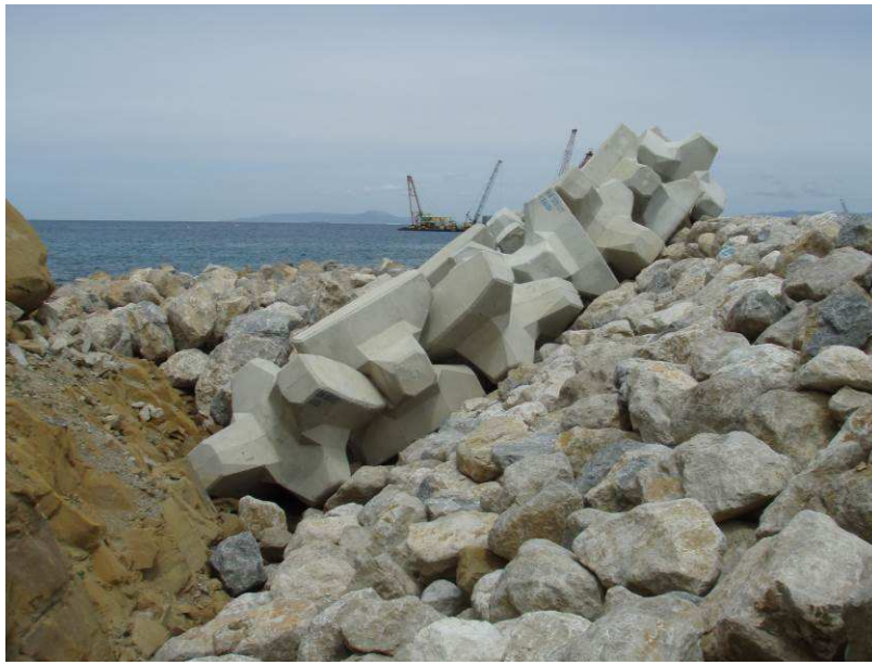
Figure 1. Construction of single layer armouring made of ACCROPODE™ units.
