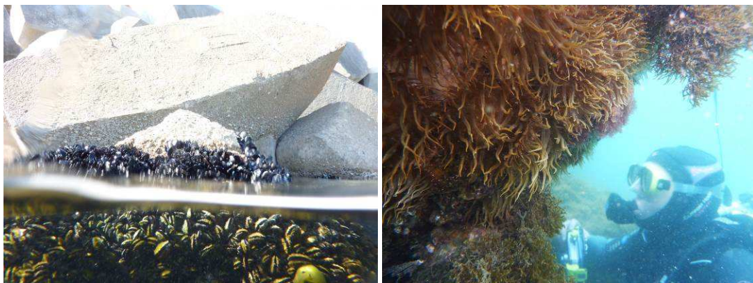
Figure 16. Mussels on the armour unit (left) and Shaded face of an armour unit colonized by anemone in the South of France (right)
