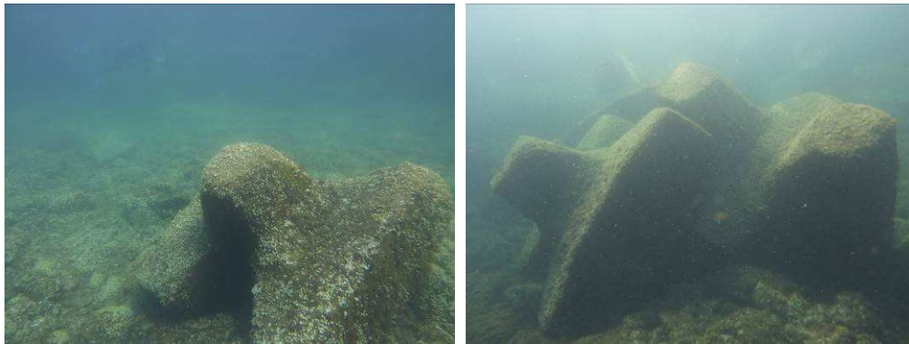
Figure 9. Single extracted unit laying on the seabed (left), group of extracted units (right).
