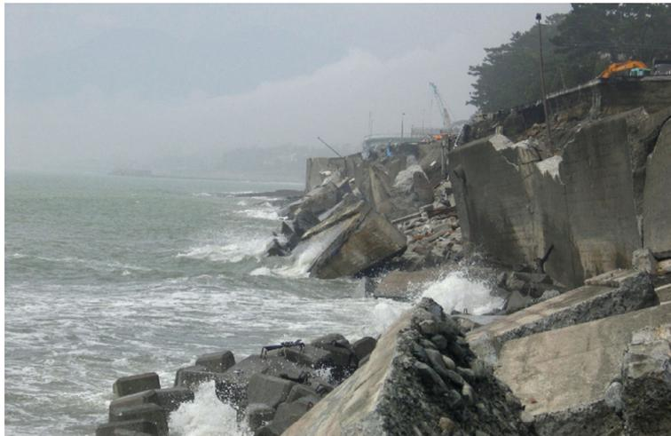
Fig. 3. Collapse of Seisho Bypass owing to storm waves associated with Typhoon 0709 hit on September 8, 2007.
