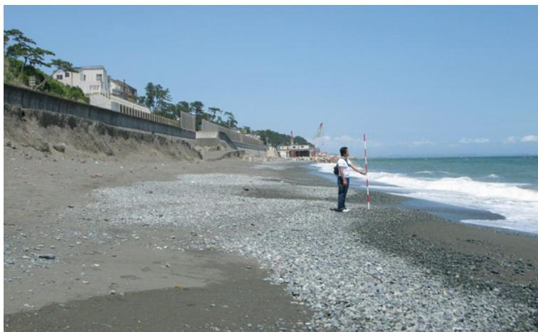
Fig. 6. Deposition of gravel on foreshore after nourishment (July 12, 2011).
