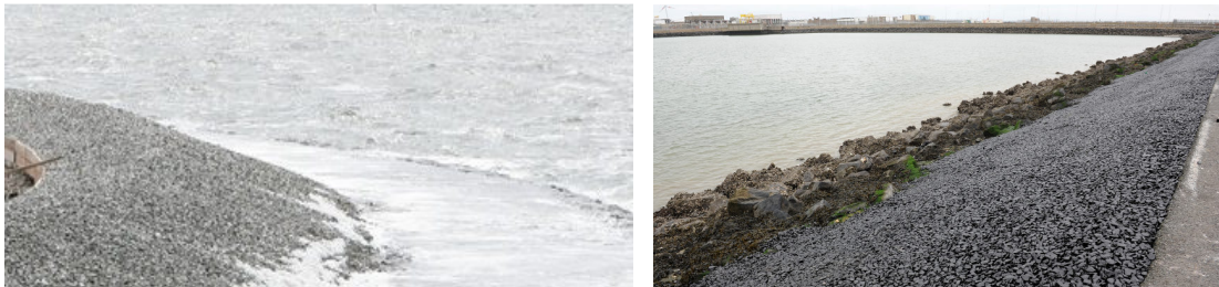
Figure 1. Detail of a porous PBA-revetment (Photos: BASF, 2013)
