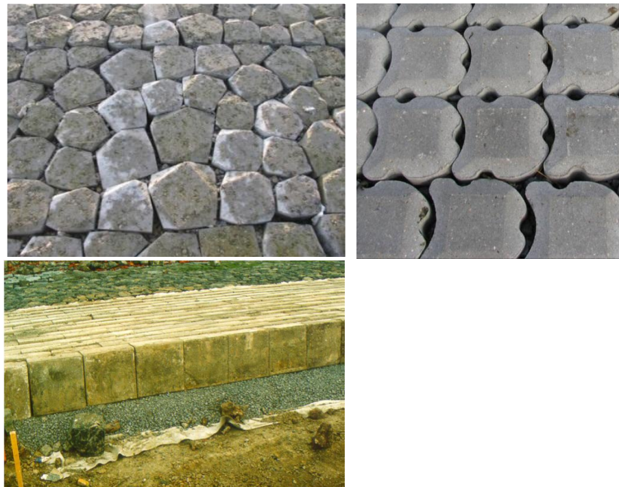
Figure 15, frequently applied types of block revetments in the Netherlands (left: Basalton; right: Hydroblocks; bottom: rectangular blocks)
