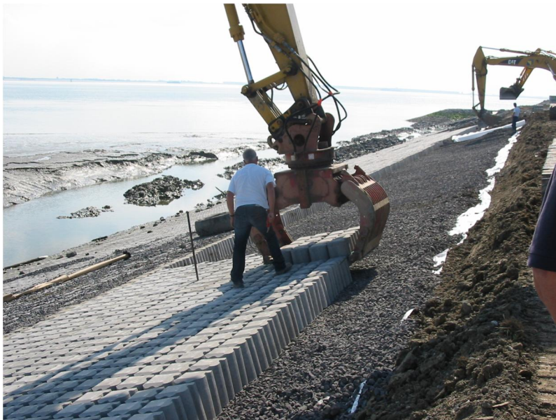
Figure 1, Block revetment during construction.
