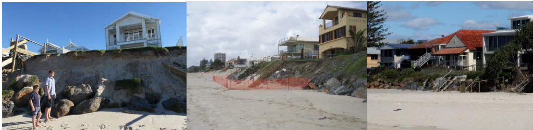
Figure 1: Examples of erosion on Palm Beach.
