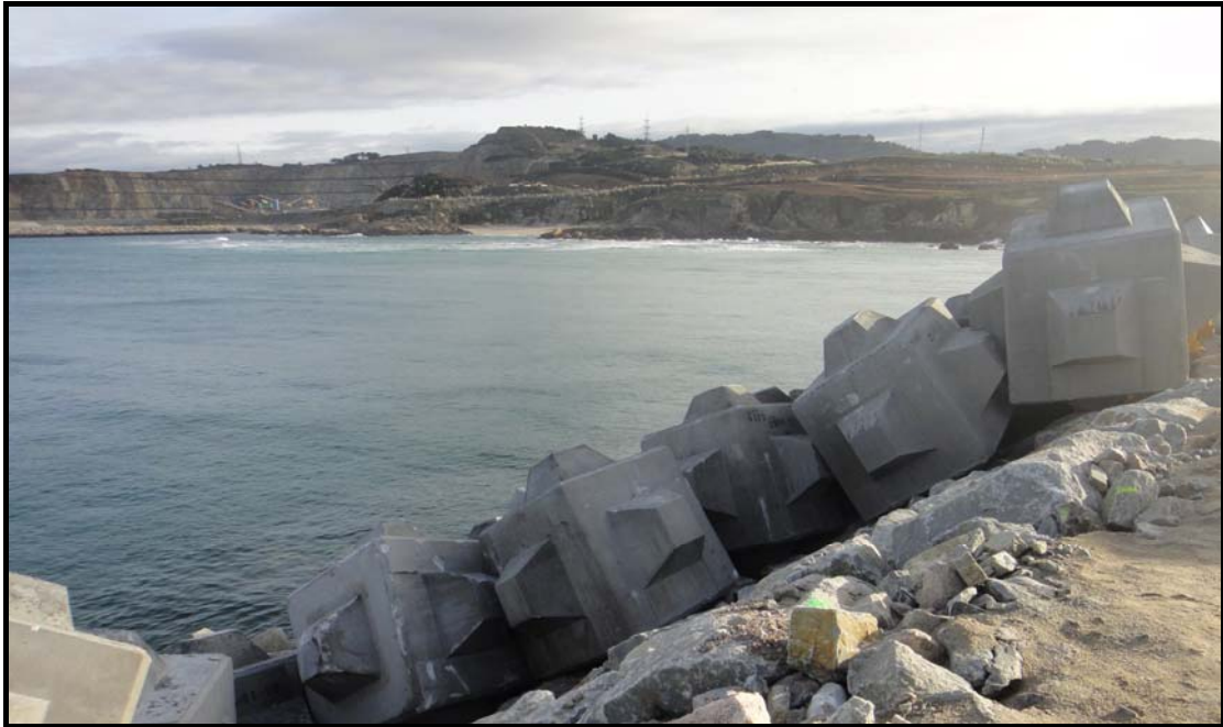
Figure 8. 15-tonne Cubipod units on the armor slope of the southern breakwater.
