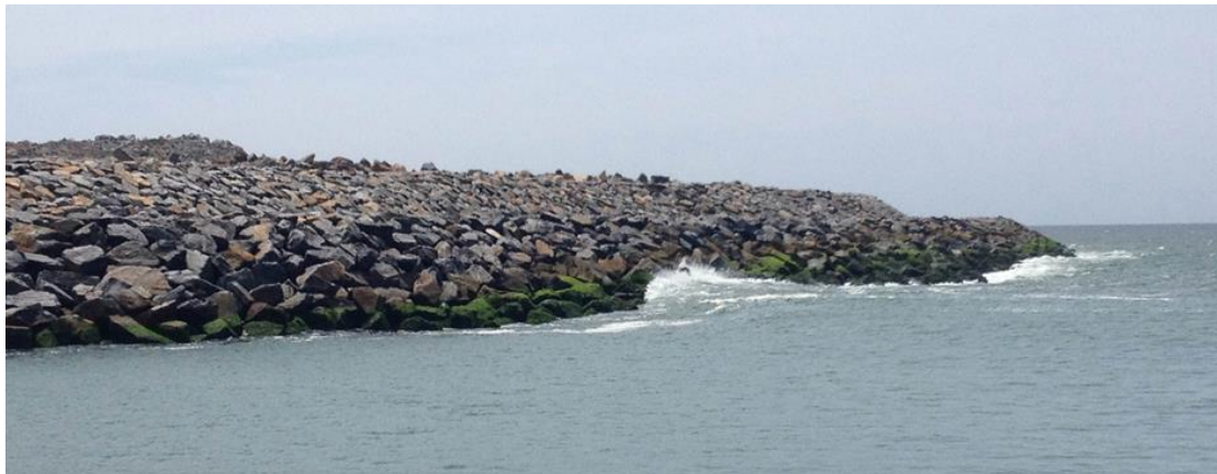
Figure 14. Fully constructed berm during the monsoon period.
