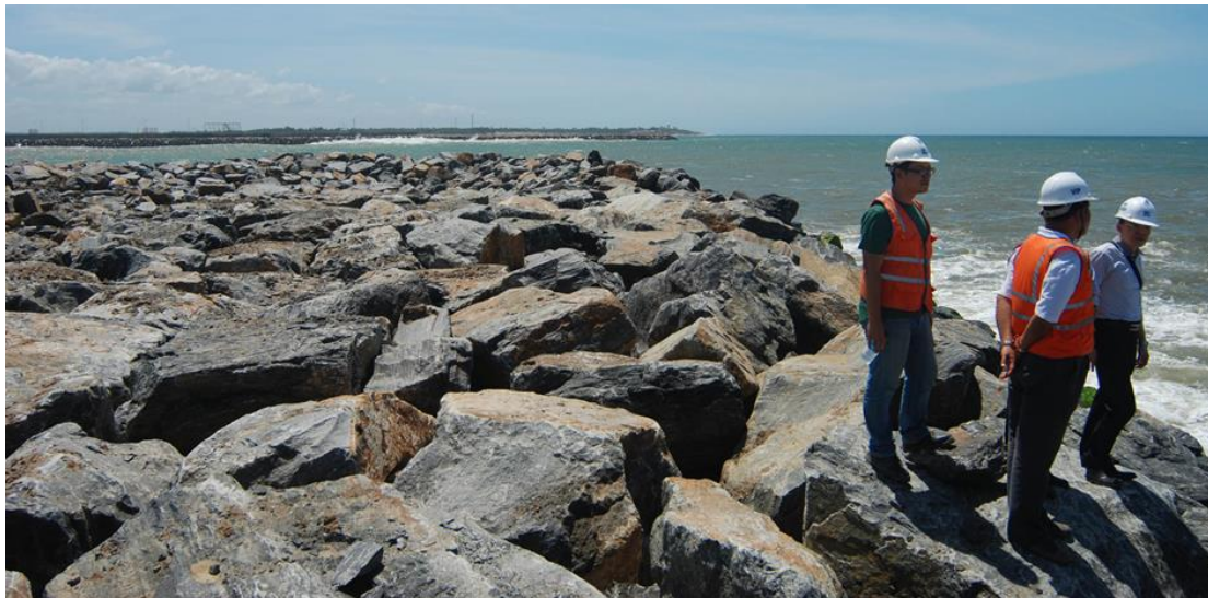
Figure 11. Partly constructed berm.
