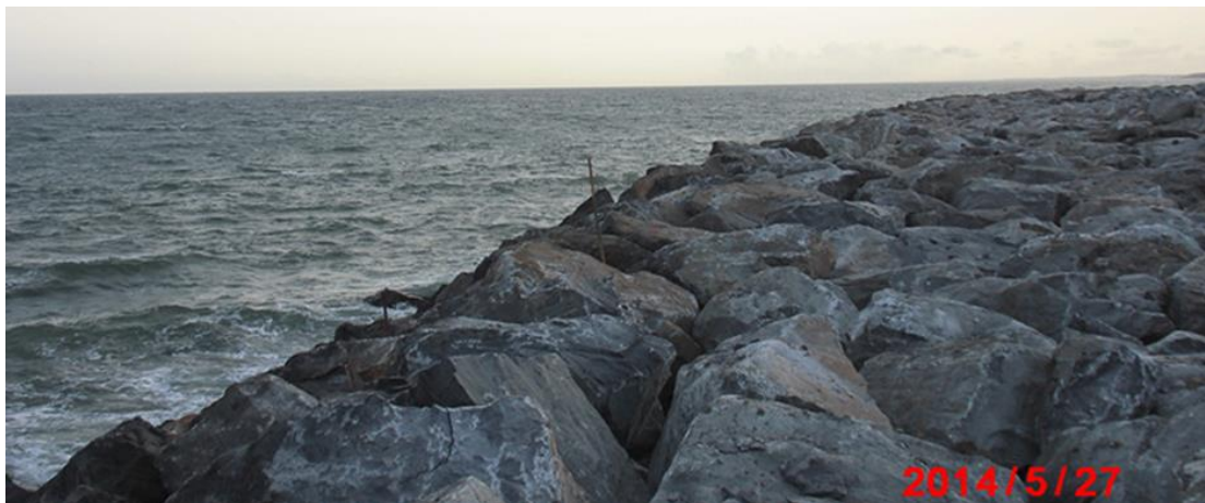
Figure 12. Fully constructed berm consisting of 5-10 tonnes rock.
