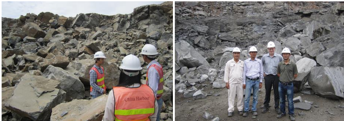
Figure 10. The FHEC team examining the blasting pile after test blasting in the harbour basin area.
