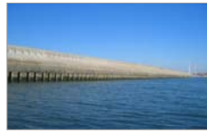
Fig. 2 Perforated breakwater in Dalian, China
