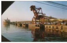
Fig. 1 Coal quaywall in Qinhuangdao, China
