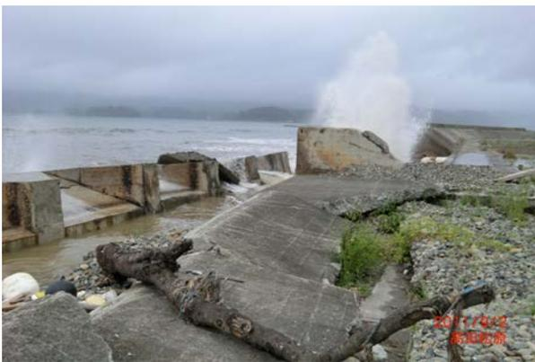
Figure 1 Collapsed seawalls due to tsunami
