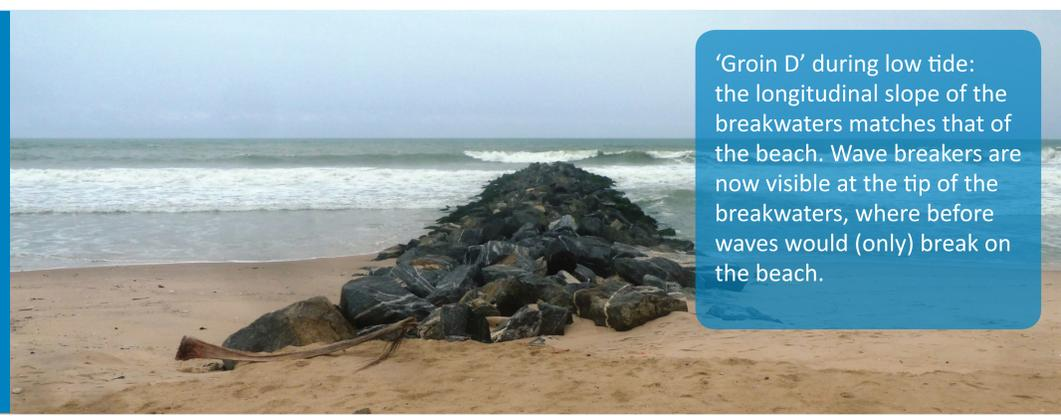
'Groyne D' during low tide: the longitudinal slope of the breakwaters matches that of the beach. Wave breakers are now visible at the tip of the breakwaters, where before waves would (only) break on the beach.
