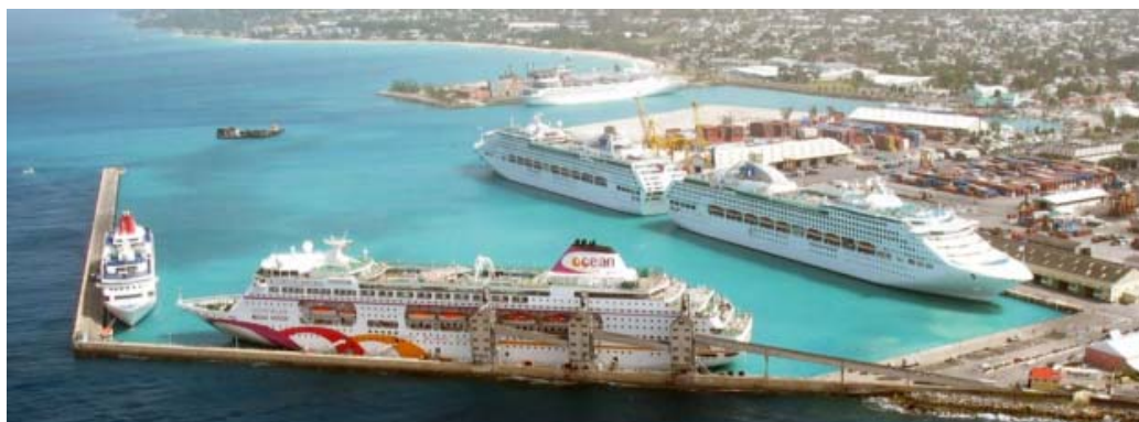
Figure 1. Existing Port of Bridgetown (photo courtesy of Foster & Ince)
