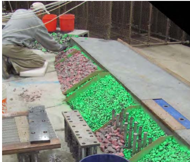
Figure 14. Construction of Armour Stone Revetment
