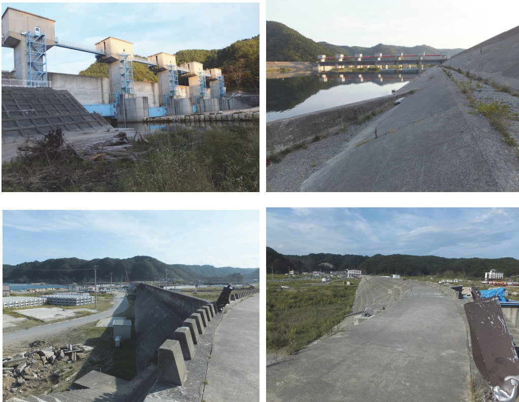
Figure 6. Snapshots of T.P.+15.5m Fudai flood gate (upper left), T.P.+12.7m Omoto flood gate (upper right), and T.P.+10m Tide Wall in Taro Coast (lower left is shoreside wall, lower right is 2nd wall ). Each pictures were taken in 2012.
