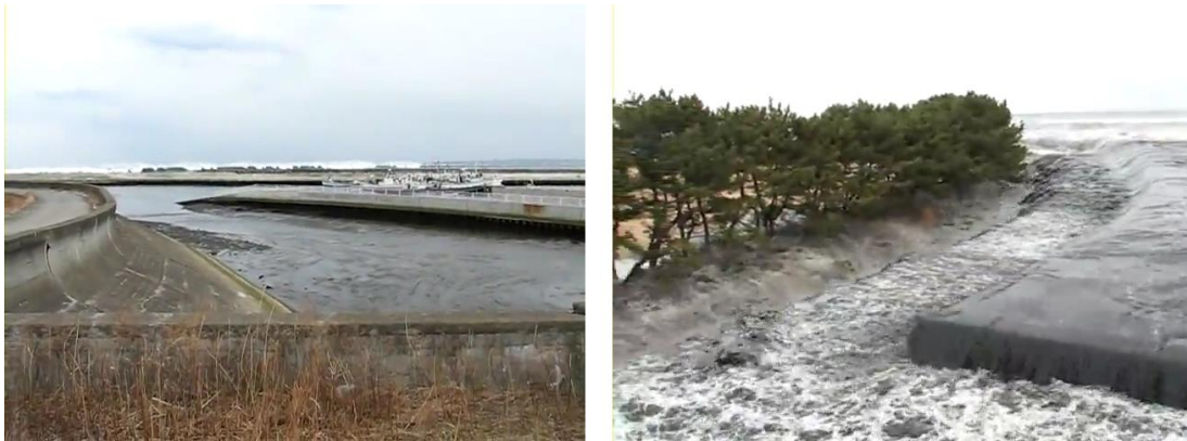
Figure 2. Snapshots of the video recorded in Oirase Town during the 2011 Tohoku Tsunami. Left one shows the approaching tsunami, and right one shows the overflowing tsunami.
