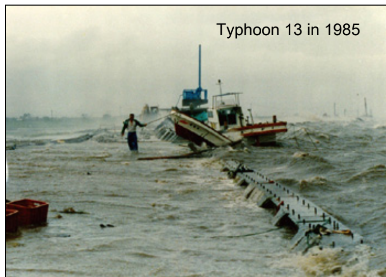
Figure 2. An example of the storm surge disasters occurred in the Ariake Sea in the past. http://www.k-keikaku.or.jp/xc/modules/pc_ktech/index.php?content_id=1791
