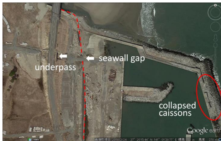
Figure 3. Damage of breakwater caissons in the Tomioka Harbor. Damage of seawalls was significant near the seawall gap connected with an underpass of a shore-parallel road embankment. The embankment appeared to be effective in reducing the tsunami force.
