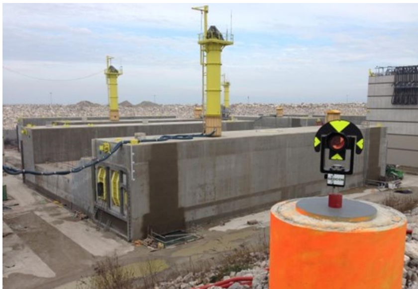
Figure 3. Gate caisson (middle) and shoulder caisson (right) ready for placement.
