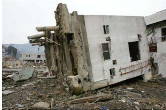
Photo 1. Structural damage due to tsunami in 2011 in Japan.
