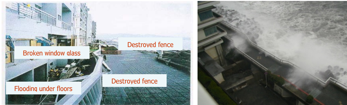
Photo 1. Serious damage caused by Typhoon in hot-spring hotel area
