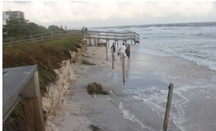
Figure 4: Dune scarping and erosion in Pinellas County immediately after Tropical Storm Debby. Photo by Hilary Stockdon, USGS, 2012.
