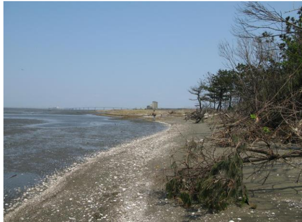
Figure 7. Concave shoreline extending from north end of L-shaped revetment.
