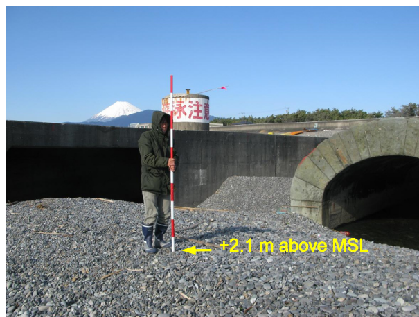
Figure 7. Berm height of 2.1 m above MSL in front of the mouth of old floodway.
