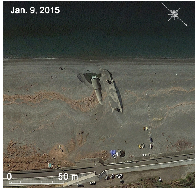
Figure 1. Satellite image of Shin-nakagawa floodway taken on January 9, 2015.
