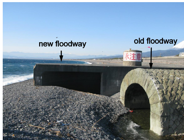
Figure 2. Horseshoe and rectangular mouths of old and new Shin-nakagawa floodways, respectively, and deposition of gravel in front of the mouths.
