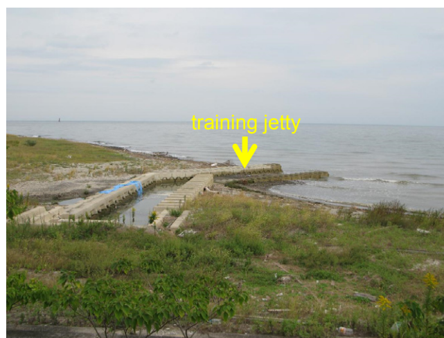
Figure 3. Training jetty extended near south end of the barrier (October 18, 2013).
