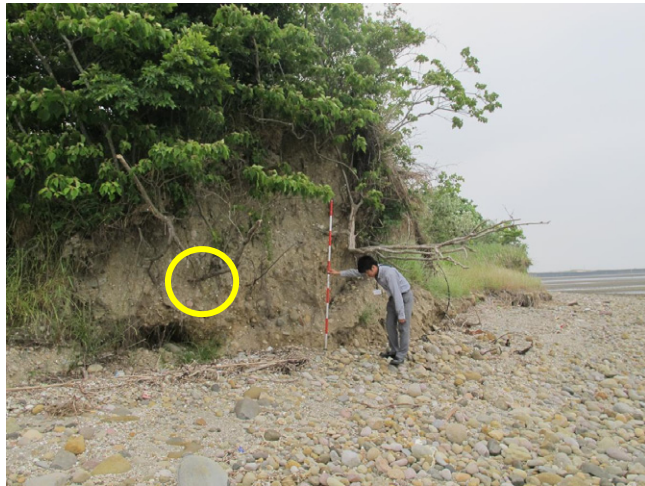
Figure 7. Scarp formed at north end of east part of artificial mound (October 18, 2013).
