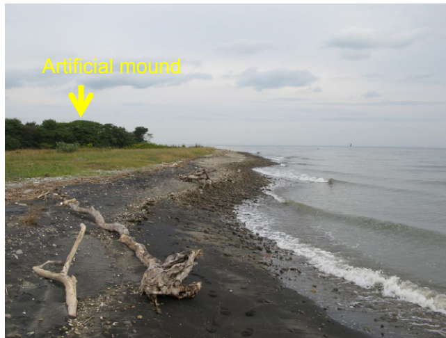
Figure 10. Oblique wave incidence immediately north of jetty (October 19, 2013).
