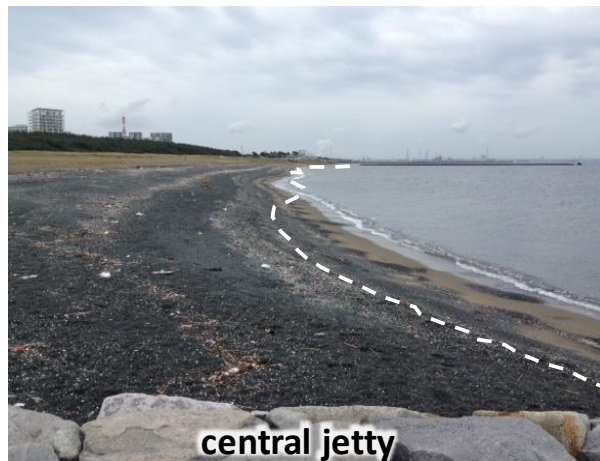
Figure 7. Changes in beach condition in area south of central jetty between May 30 and October 8 in 2012.
