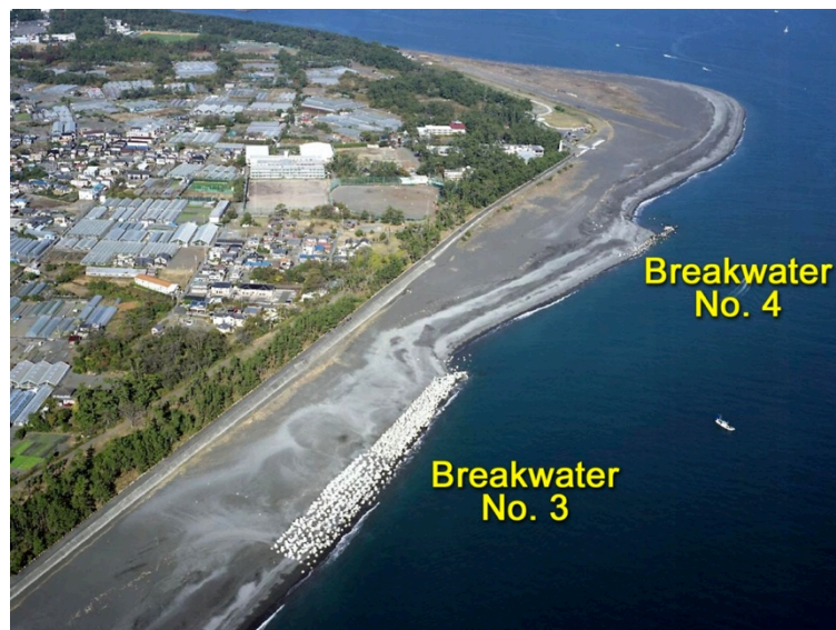
Figure 7. Oblique aerial photograph between BW3 and BW4.
