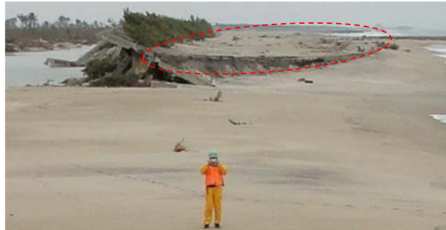
Figure 5. Erosion of beach adjacent to the breaching after the tsunami (cliff beach) (Taken: April 2, 2011)
