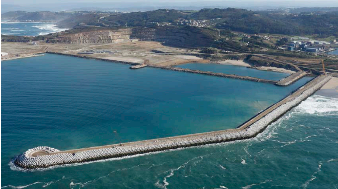
Figure 12. Western Breakwater during construction (October 29 th , 2015).
