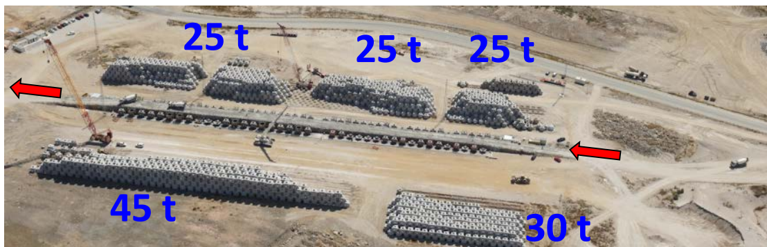
Figure 7. Aerial view of the Cubipod ® block yard (July 7 th , 2015)
