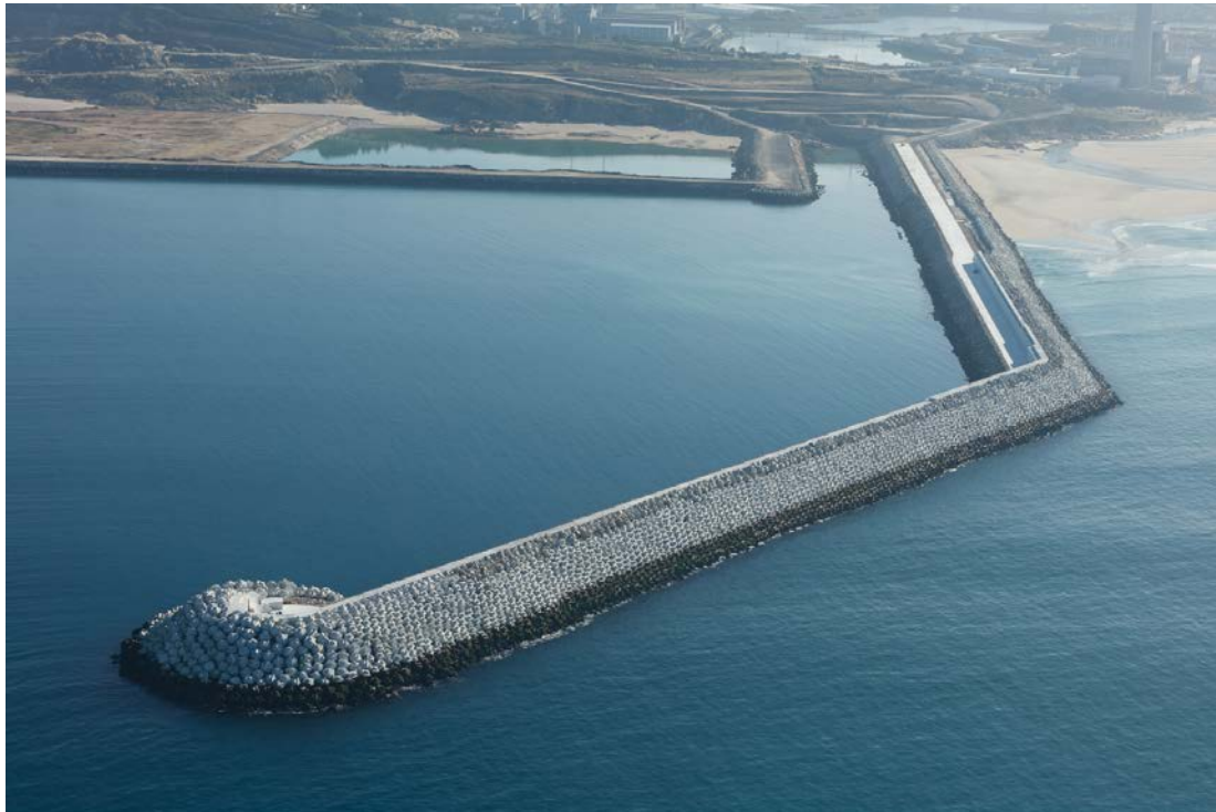
Figure 13. Western Breakwater (November 16 th , 2016).
