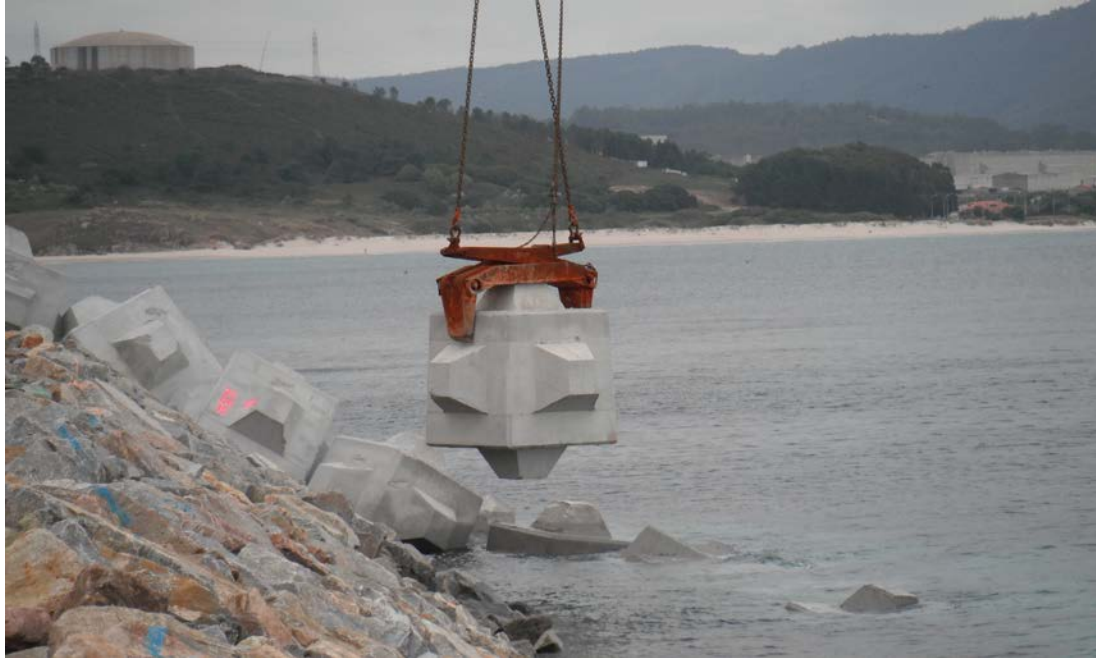
Figure 10. Placing 25-tonne Cubipods in the Western Breakwater.
