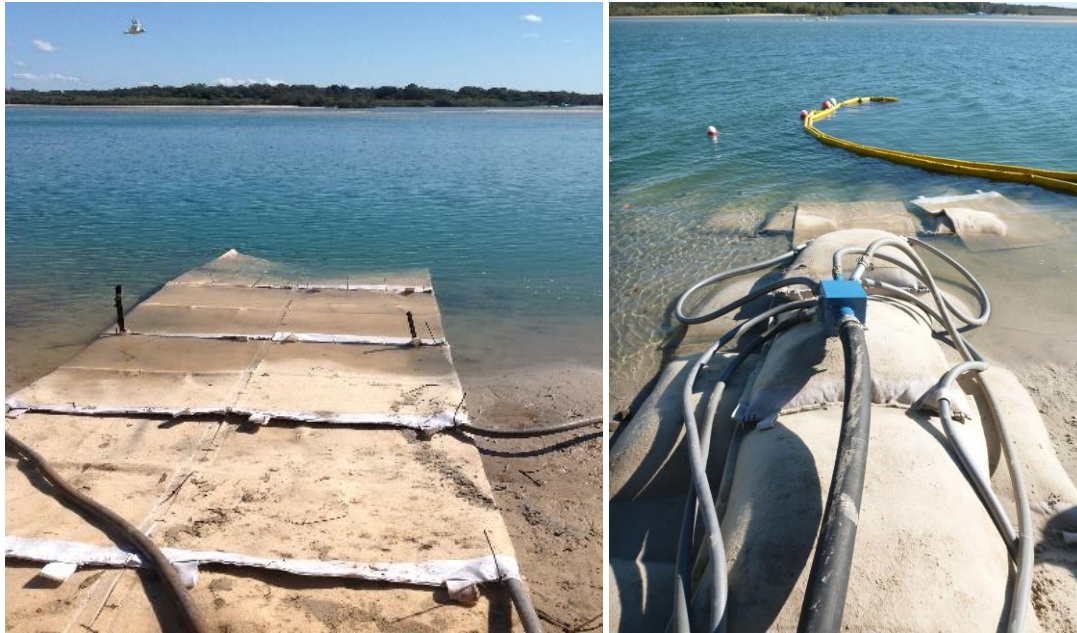
Figure 8. Novel Method of Filling Sand-Filled Geotextile Containers In-Situ
