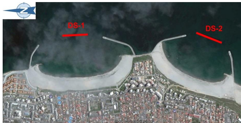
Figure 2 Location of the submerged breakwaters within the coastal protection system (DS-1 in Tomis North area and DS-2 in Tomis Centre area)
