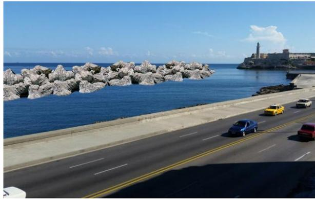
Figure 21. View of the LCB with concrete units with a large degree of interlocking.
