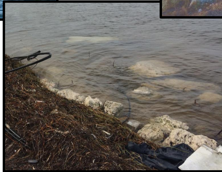
Revetment: armament displaced
