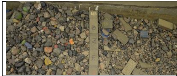
Figure 3 Example collapsed breakwater
