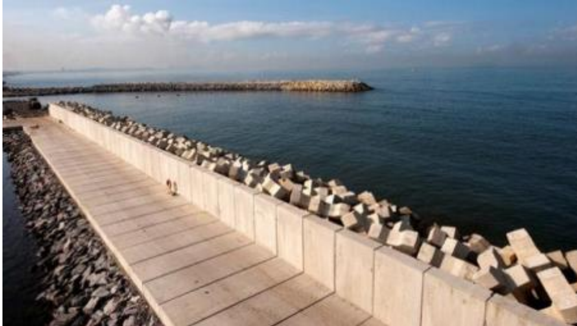
Crown wall on top of a breakwater at Dikkowita Port ( www.xbloc.com )
