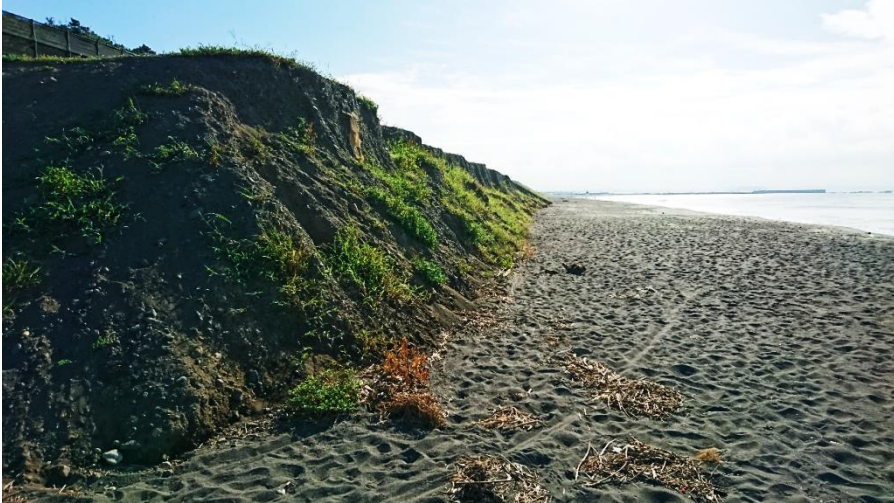
Figure 2. Sand mound for beach nourishment in Yanagishima area (August 16, 2016).
