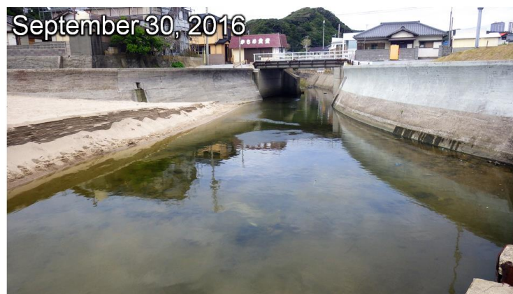
Figure 8. Raised water level owing to backwater effect caused by river mouth closure.
