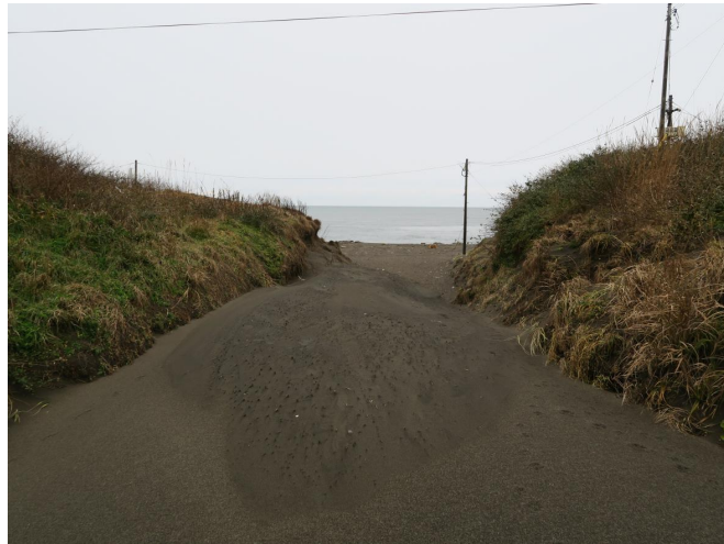
Figure 12. Sand deposition at landward entrance to coast (November 3, 2016).
