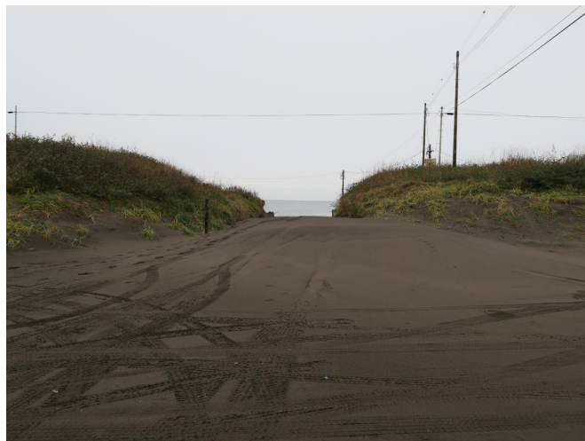
Figure 13. Sand deposition around entrance of beach access (November 3, 2016).
