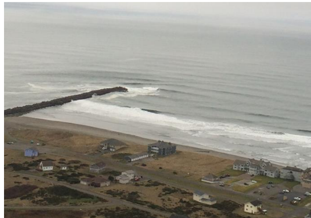
Figure 1 - Grays Harbor North Jetty on the Pacific Ocean
