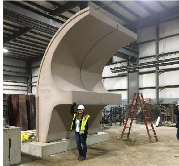
Figure 1 - Precast Individual Wall Sections
