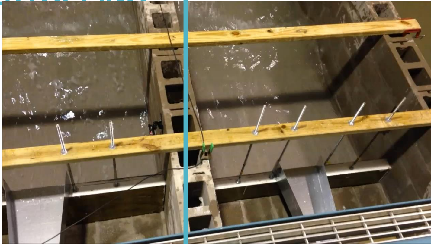
ELEVATION +16 FT ECD (9.0 FT WALL ABOVE ROAD) ELEVATION + 12 ECD (5.0 FT WALL ABOVE ROAD) NOTE OVERTOPPING OCCURS AT BOTH WALL HEIGHTS
