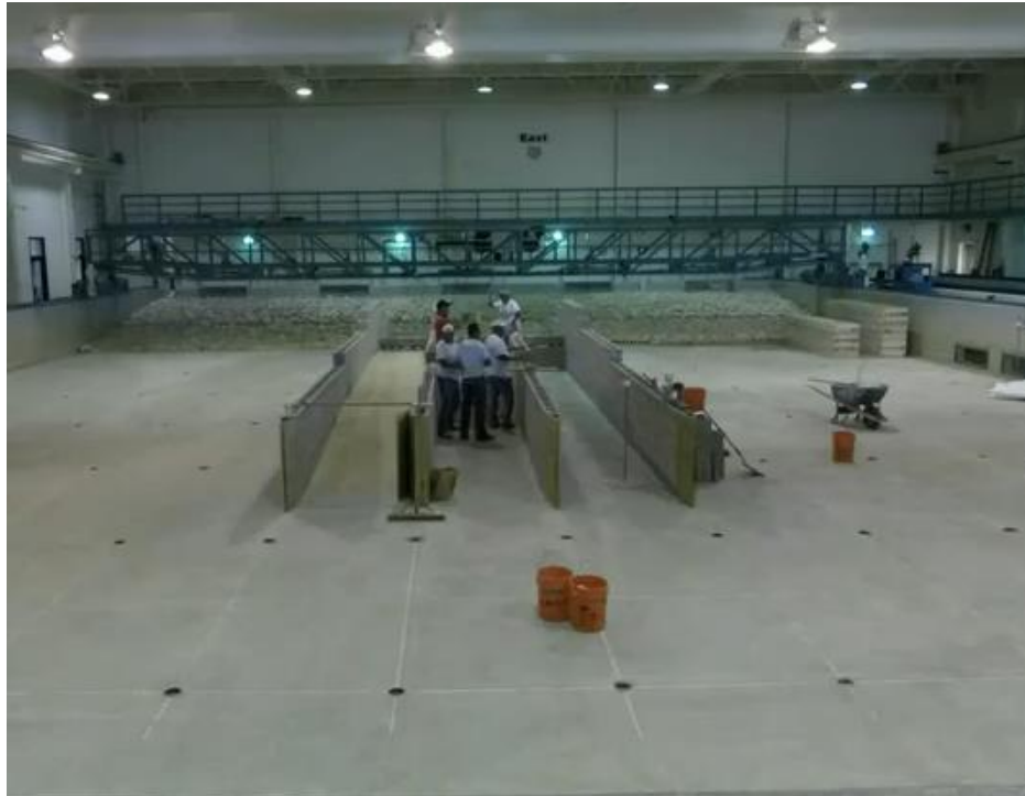
PLACING SAND BEACH
