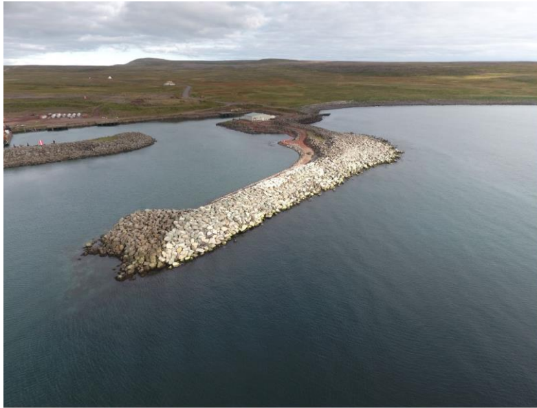
Figure 6. Aerial photograph of completed Phase 1 repairs. (Photo courtesy of Brice Construction).
