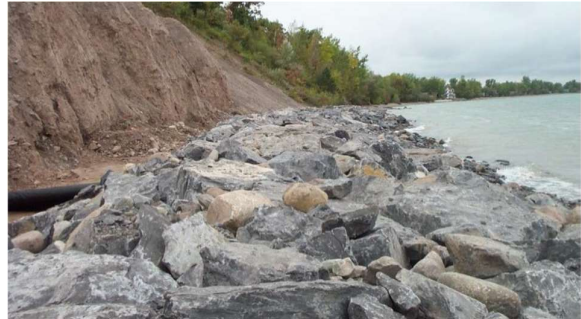
Figure 2 - Armor Stone Installed at the Toe of the Bluff
