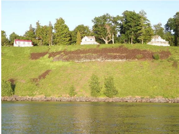
Figure 5 - Slope Repairs along the Groundwater seepage Line.
