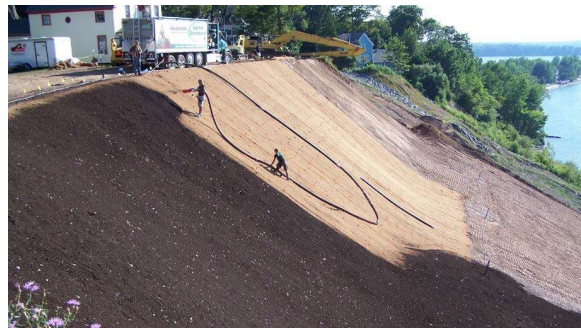
Figure 3 - Installation of the Veneer Cover System
